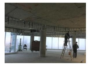
These photos feature the steel stud framing for the curved bulkheads, above the Metro Vancouver boardroom and audience seating areas. These bulkheads are curved to the radius of the boardroom table and the tiered seating.
